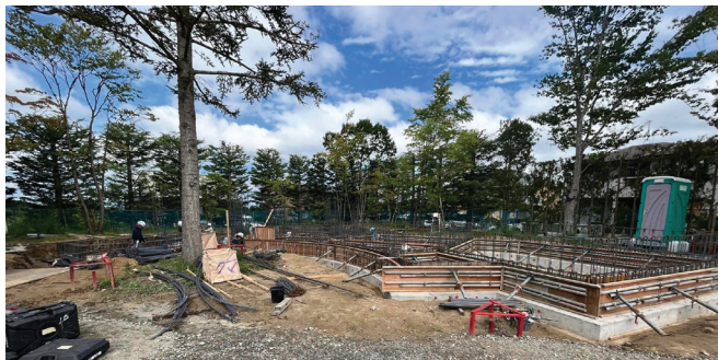
Earthquake-proof foundation of the new Funehiki church
