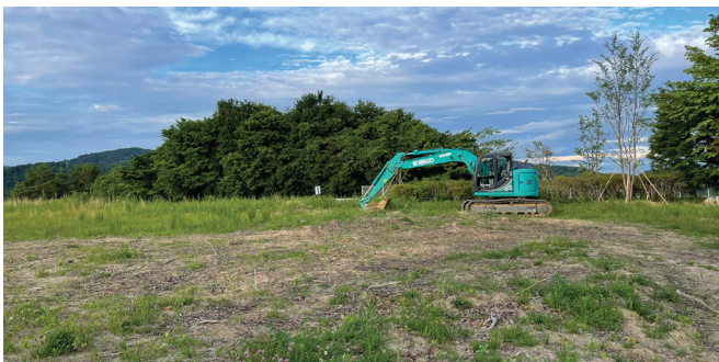
Church site after clearing of trees
